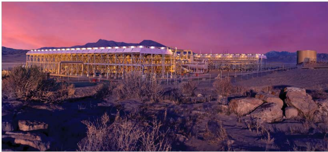
Salt Wells geothermal plant in Nevada. Photo: U.S. Department of Energy
